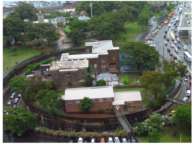
Photo 1| Existing School Site Source: A View of Sydney
